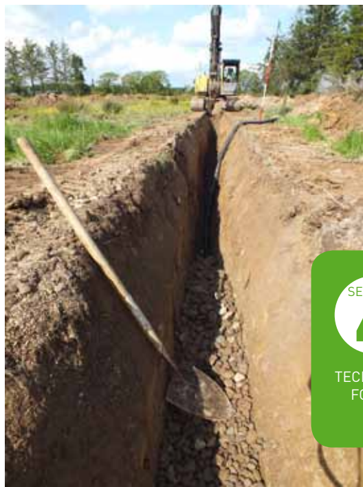
Figure 2. Drainage trench excavation
