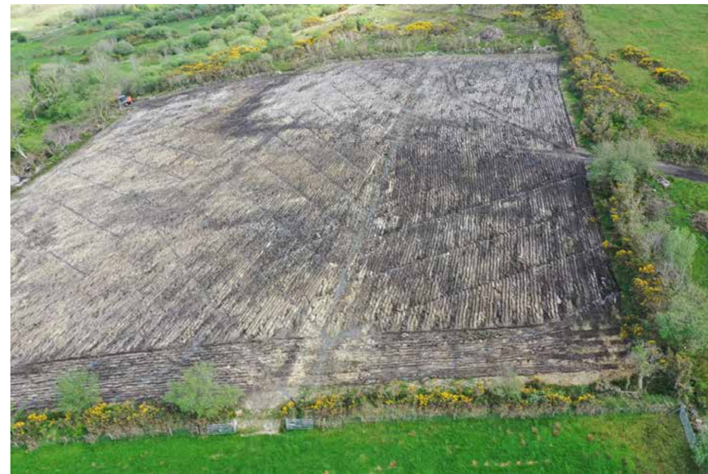
Aerial photo of drainage works pre reseeding
